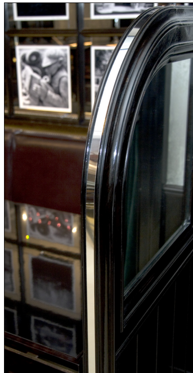
Detail of the bar's privacy wall, which is constructed of ebonized walnut, polished stainless steel, and glass.
