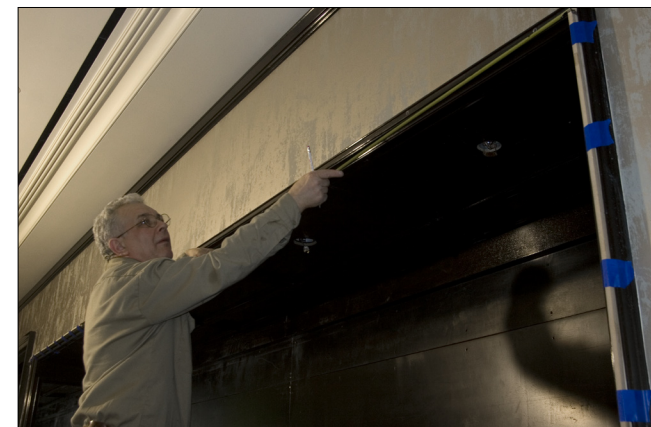
Installation of case molding wall panels.
