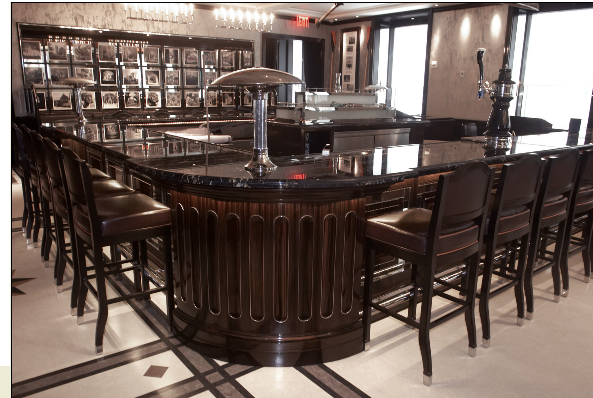
Details of the bar corner constructed of solid lumber and veneer in macassar ebony. The bar corners contain metal insets with fluted details. A custom-made lamp is recessed into the black portoro marble counter.
